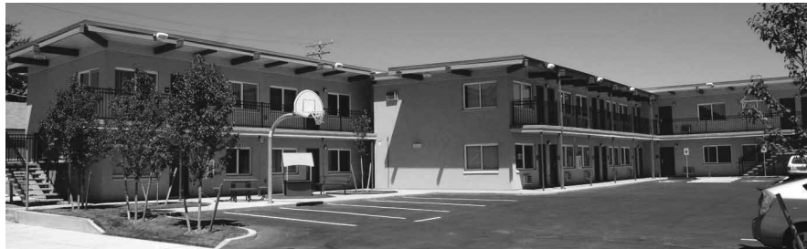
La Posada East and West have dormitory-style rooms for single individuals as well as family rooms. The total capacity is over 200 residents. Photo by Ricardo Sanchez, courtesy of Sea Mar Community Health Center
