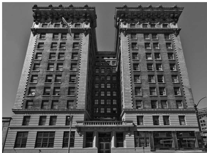
The Frye Hotel was built by Seattle pioneer George F. Frye and his wife Louise (Denny) Frye, in 1911. The hotel was purchased and restored in 1997 as housing for low-income and formerly homeless persons. Photo courtesy of W.G. Clark.
